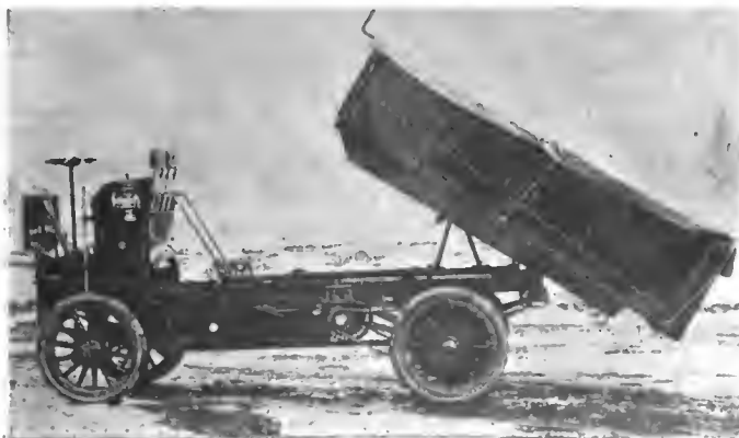
KNOX DUMPING ASH WAGON FOR THE CITY OF CINCINNATI.
